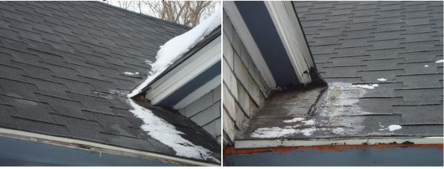
Areas of leakage are in the valleys (and below the valleys) adjacent to the south dormer, and the upper ridge area of the dormer.
